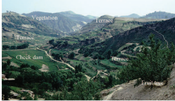
Figure 14: Combination of soil conservation measures at Yan'an site in the Loess Plateau, China
